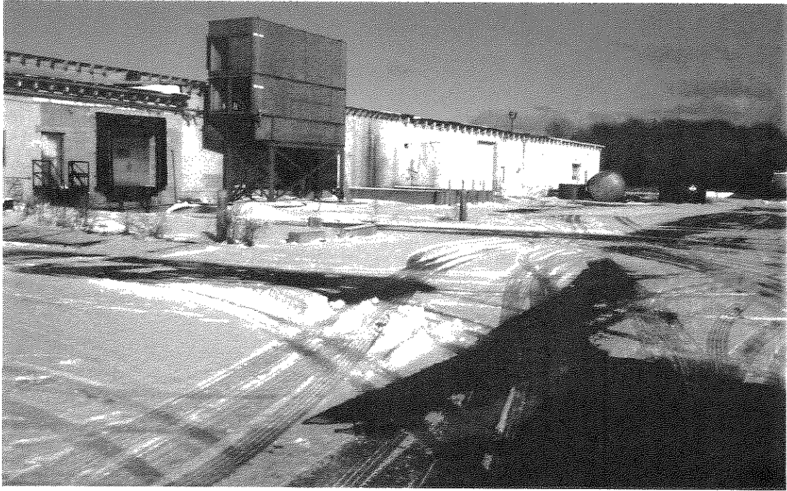
BECHTEL-MCLAUGHLIN: SOUTH EXTERIOR
